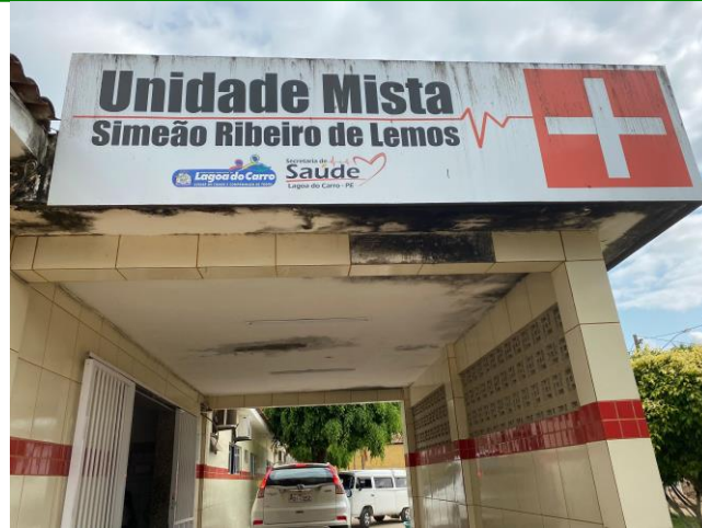
35.16. Fachada do Hospital
