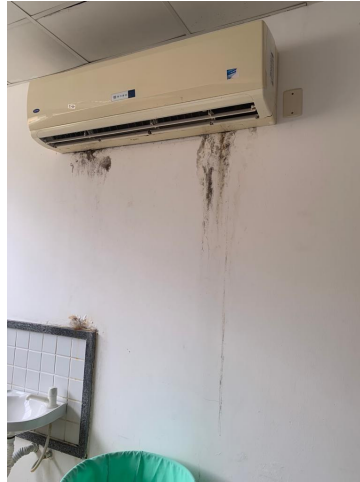
40.63. Split e Mofo
